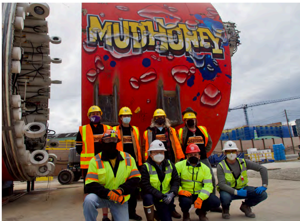
MudHoney, the 18 foot diameter Tunnel Boring Machine, and crew will build the conveyance tunnel for the Ship Canal Project. (Image courtesy of Seattle Public Utilities.)
