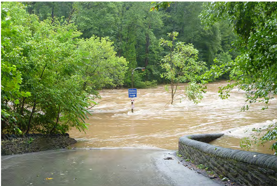
Flooded roadway in Philadelphia. (Photo courtesy of Philadelphia Water Department.)
