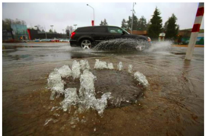
Figure 17. Overflowing stormwater, Seattle. (Photo Courtesy of Seattle Public Utilities.)
