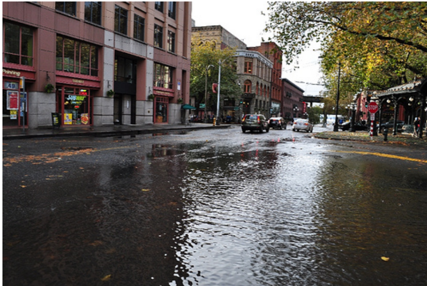
Figure 2. Flooding in Pioneer Square, Seattle, WA. Atlas 14 precipitation projections are not available in the Pacific Northwest, forcing Seattle and other Pacific Northwest cities to plan using outdated information. (Photo courtesy of Seattle Public Utilities.)
