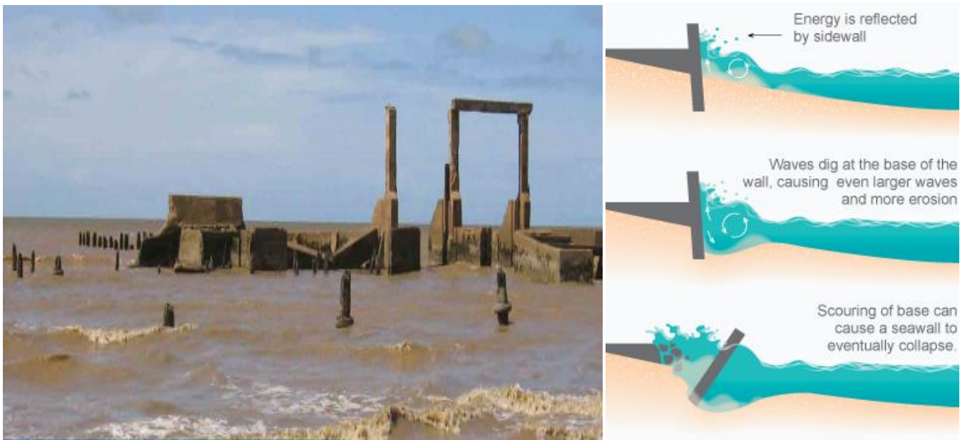
Figure 8. Failure of hardened sea defense structure in Guyana
